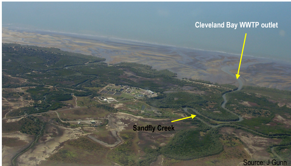
Figure 7.2 Cleveland Bay WWTP Outfall Low Tide
